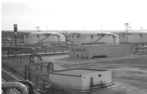
Figure 2. Shore tanks of oil terminal.
