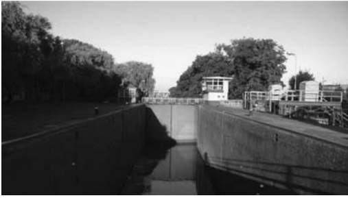
Figure 1. The lock in Czyżykówko on Wisła – Odra waterway.
