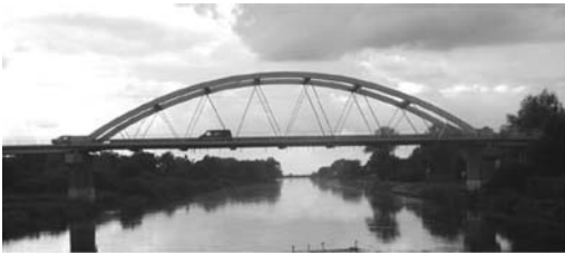
Figure 3. The road bridge over Noteć river in Santok (Poland)-(Nadolny G. 2005).
