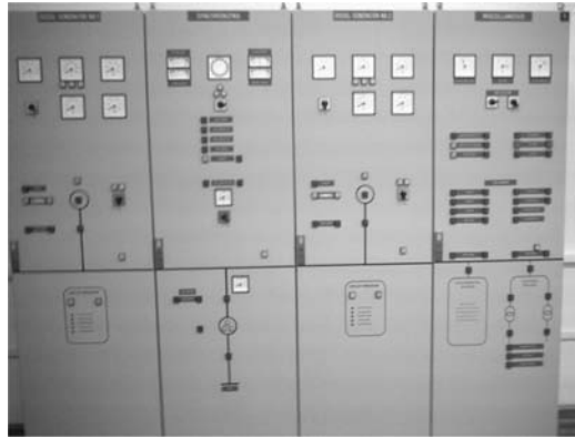
Figure 2. Main switchboard.
